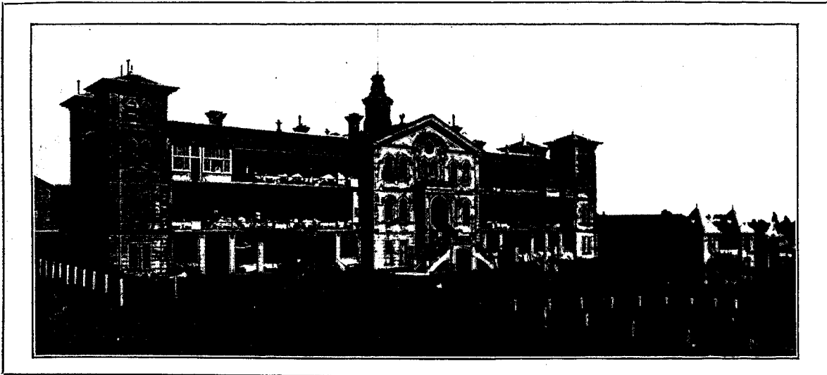
THE AUCKLAND HOSPITAL, NEW ZEALAND. MAIN BLOCK.
